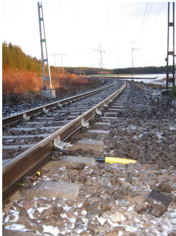
Figure 16: Sensor positions in track.
