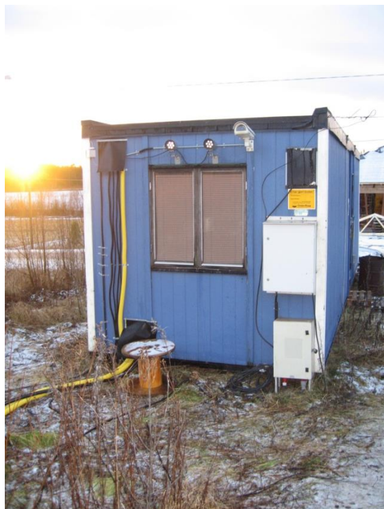
Figure 18: 2-room heated bungalow for computer and communication electronics.
